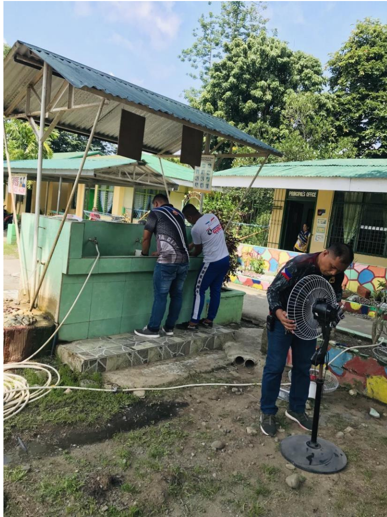
Community Extension: Brigada Eskwela cleaning of stand fan from classrooms and checking of all electrical outlets.
